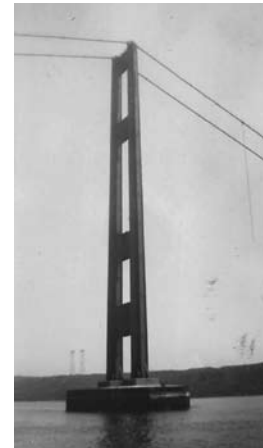
The north and south towers were all that remained of the bridge until it was rebuilt and opened in 1950. Dad took this photo from the hastily re-instituted Gig Harbor ferry in 1941.
